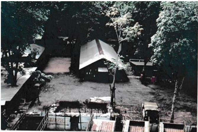
Photo taken from the water tower.
