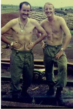
Macca and Bluey Healey take a break during the construction of 31 Delta Mk 2 at the 2/35th Artillery Battalion gun park. July-Aug 1968
