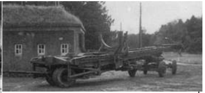
The Meillerwagen was used to transport the V2 to the firing site and used to raise the rocket.
