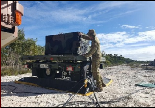
GNR Ryan Kearney – assisting with the emplacement of the 10kVa generator.
