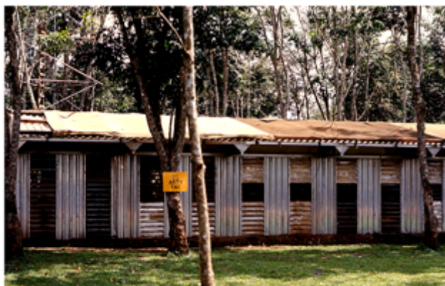
Artillery Tactical H.Q. (Arty Tac) external view 1 ATF Nui Dat 1967 note tarpaulins on roof to deaden sound of heavy rain during wet season
