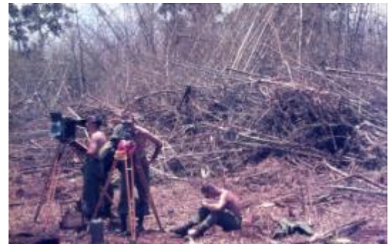
.On the right: Mick Delaney on tellurometer, Rick Mahoney on Theodolite and Jock Gunn booking.
