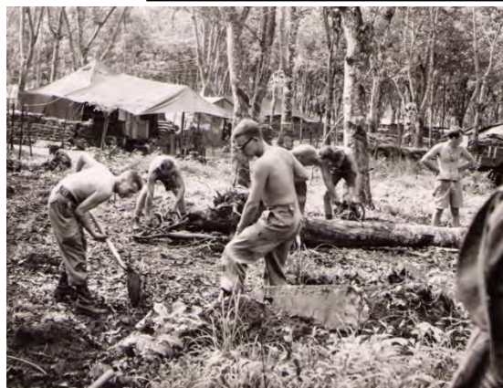
Clearing and cutting activities - L to R: Trevor Waghorn, Ray Hutchinson, Stuart Sporn, X, Roger Long and Jim Hogno supervising again
