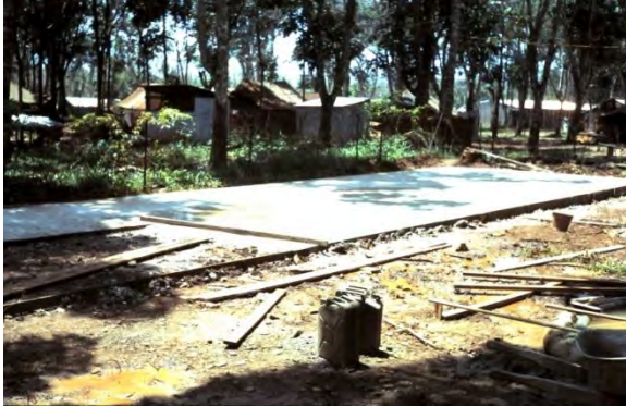
Slab farthest away from the road. Note the HQ throne room in the background, sensitively camouflaged by bushes
